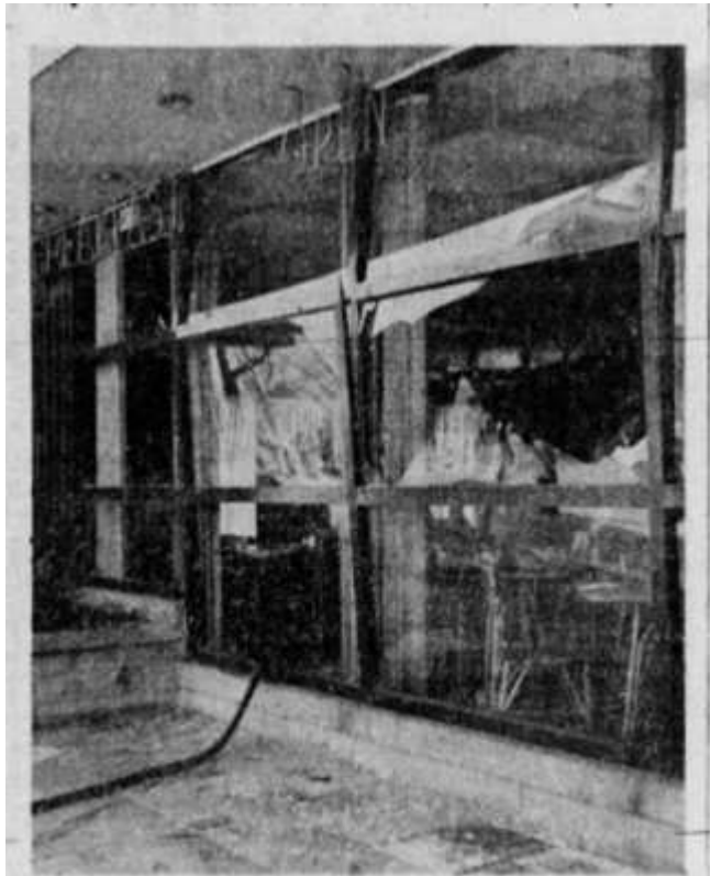
FRONT VIEW of the restaurant shows that the heavy wooden sash was bulged and broken and many of its plate-glass windows shattered by blast. Other employees on duty and about a dozen customers were unhurt.
